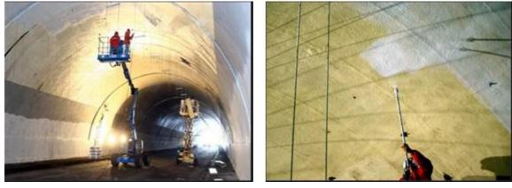
Figure 8 – Painting of the tunnel
