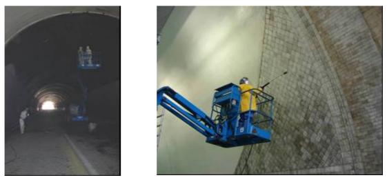
Figure 7 – Washing and cleaning of the vault
